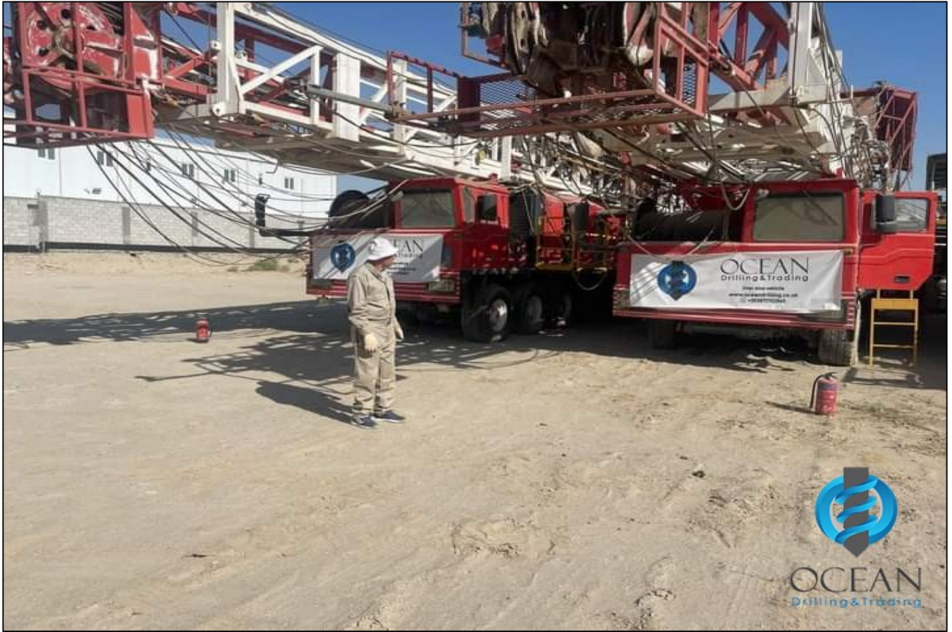
drilling rig 750hp
