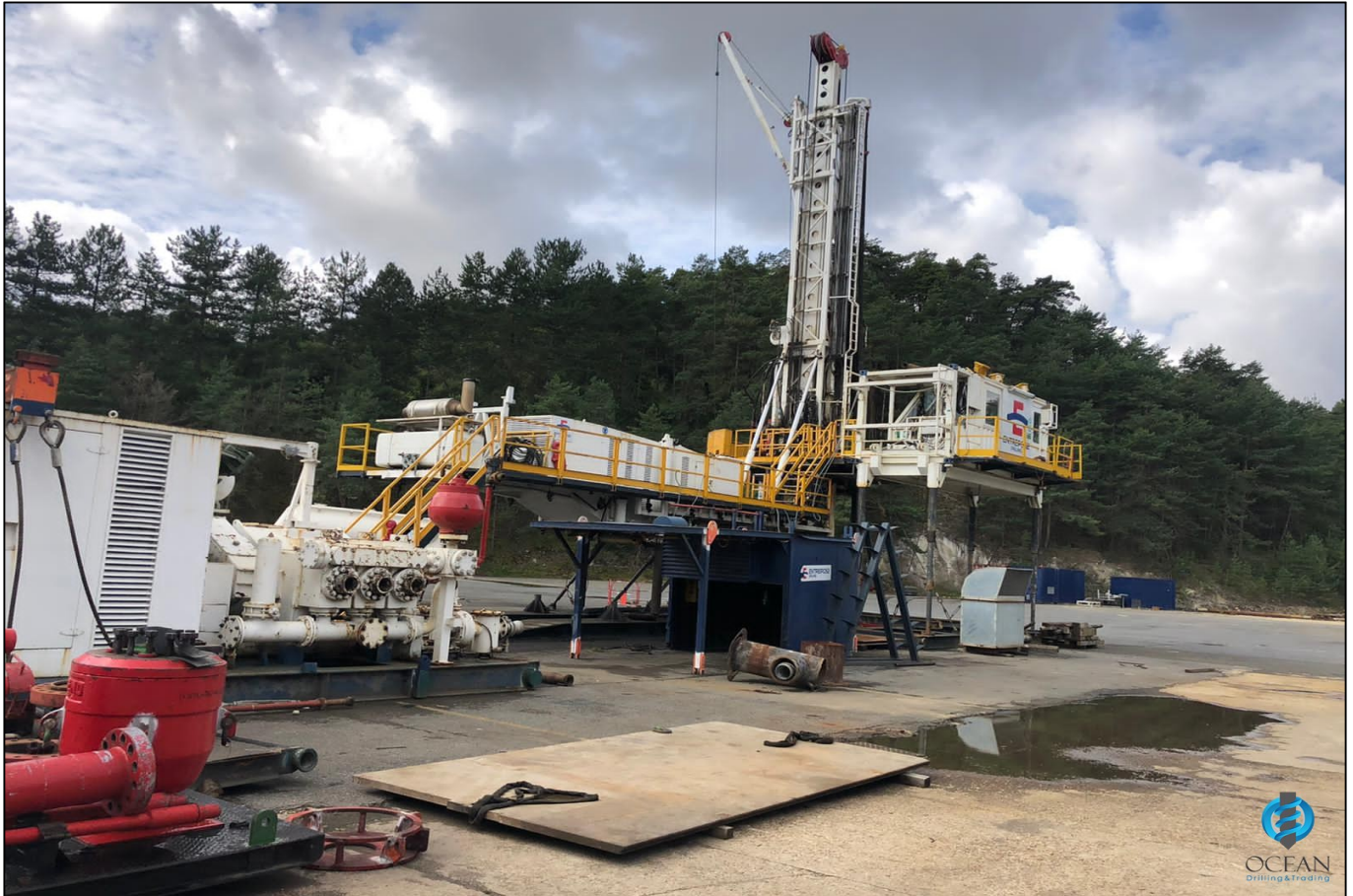
DRILMEC Drilling Rig 270 ton pull back With all equipment ready for job
