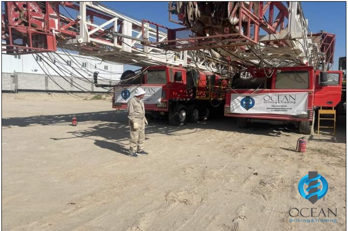
drilling rig 750hp
