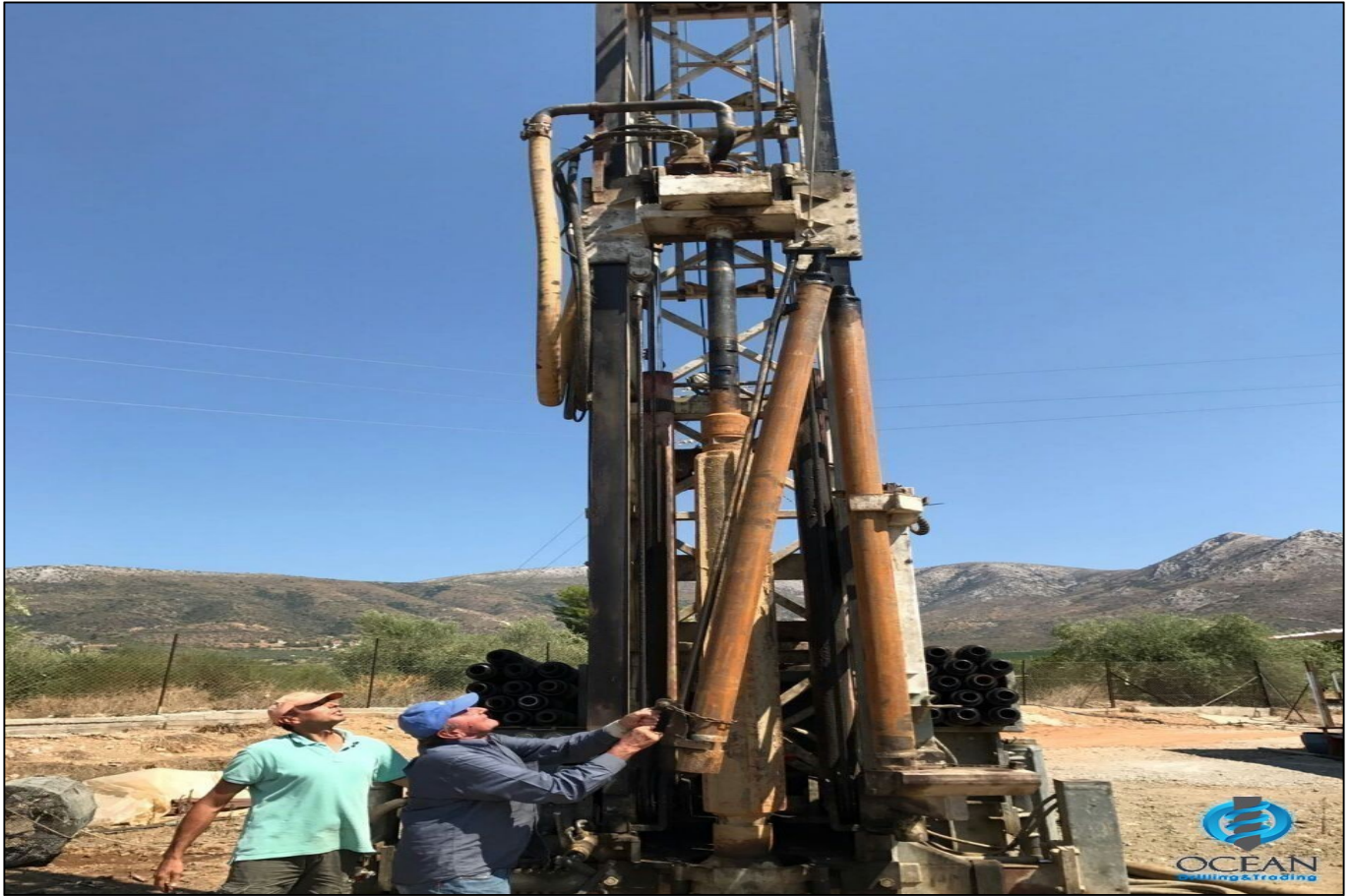
A European drilling rig
