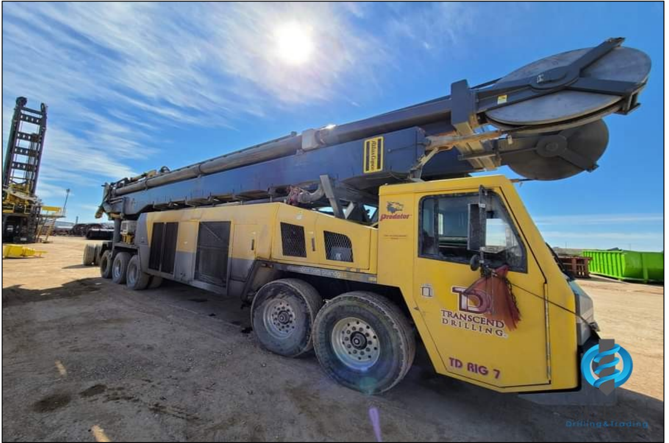
Atlas Copco drilling
